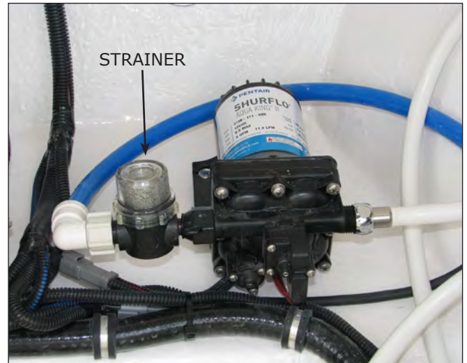
Fresh Water Pump and Strainer
