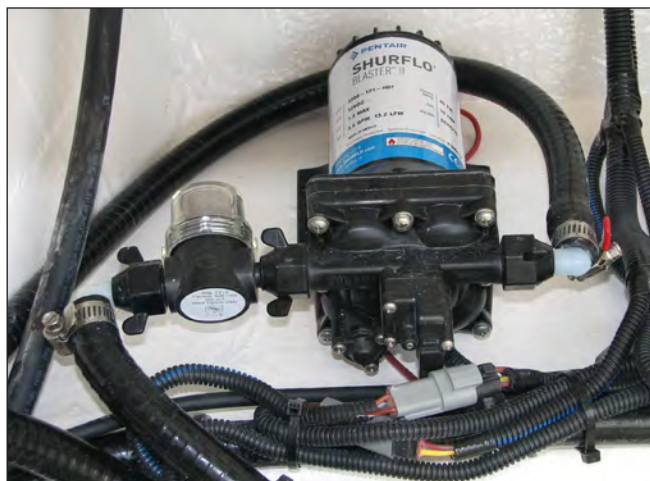
Raw Water Washdown Pump & Strainer
