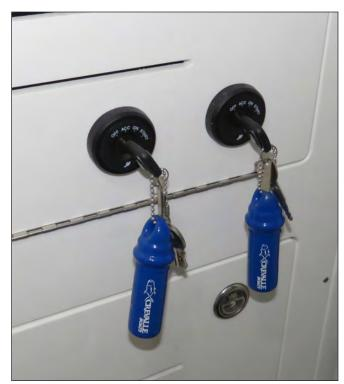
Typical Mercury ON/OFF Key Switches
